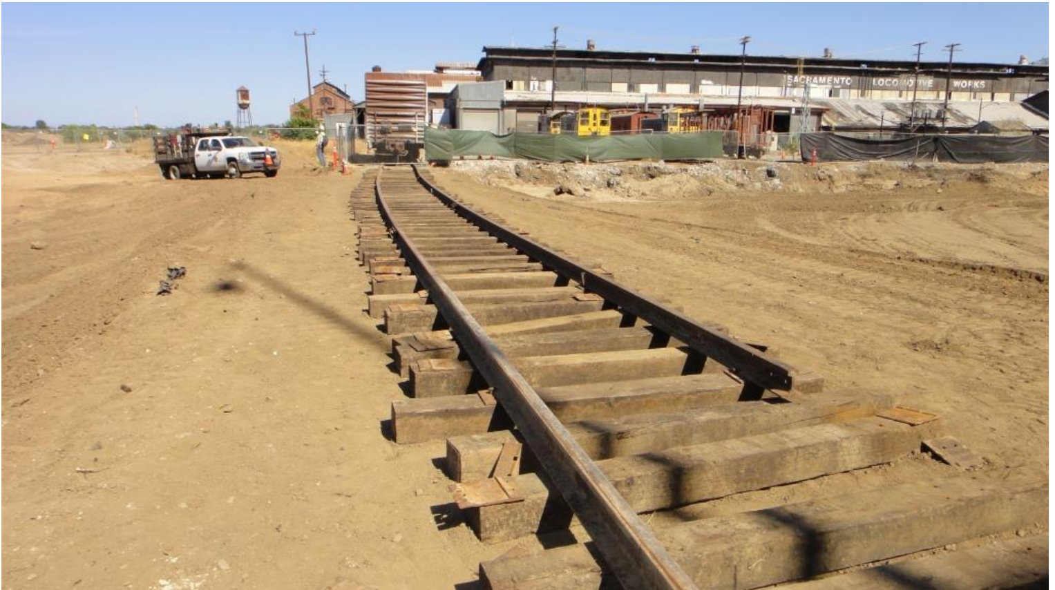
By the end of the day, there was about 120 feet of track where none had been in the morning...
