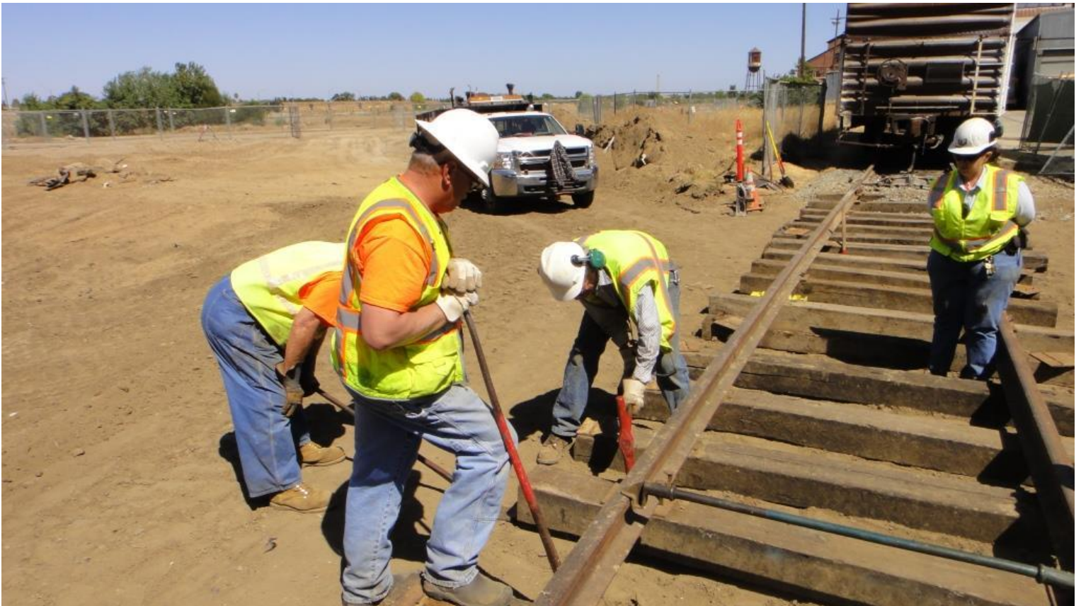
With the rails in gauge, our world-famous "as seen on TV" spiker, Steve was pounding down spikes with all his might...
