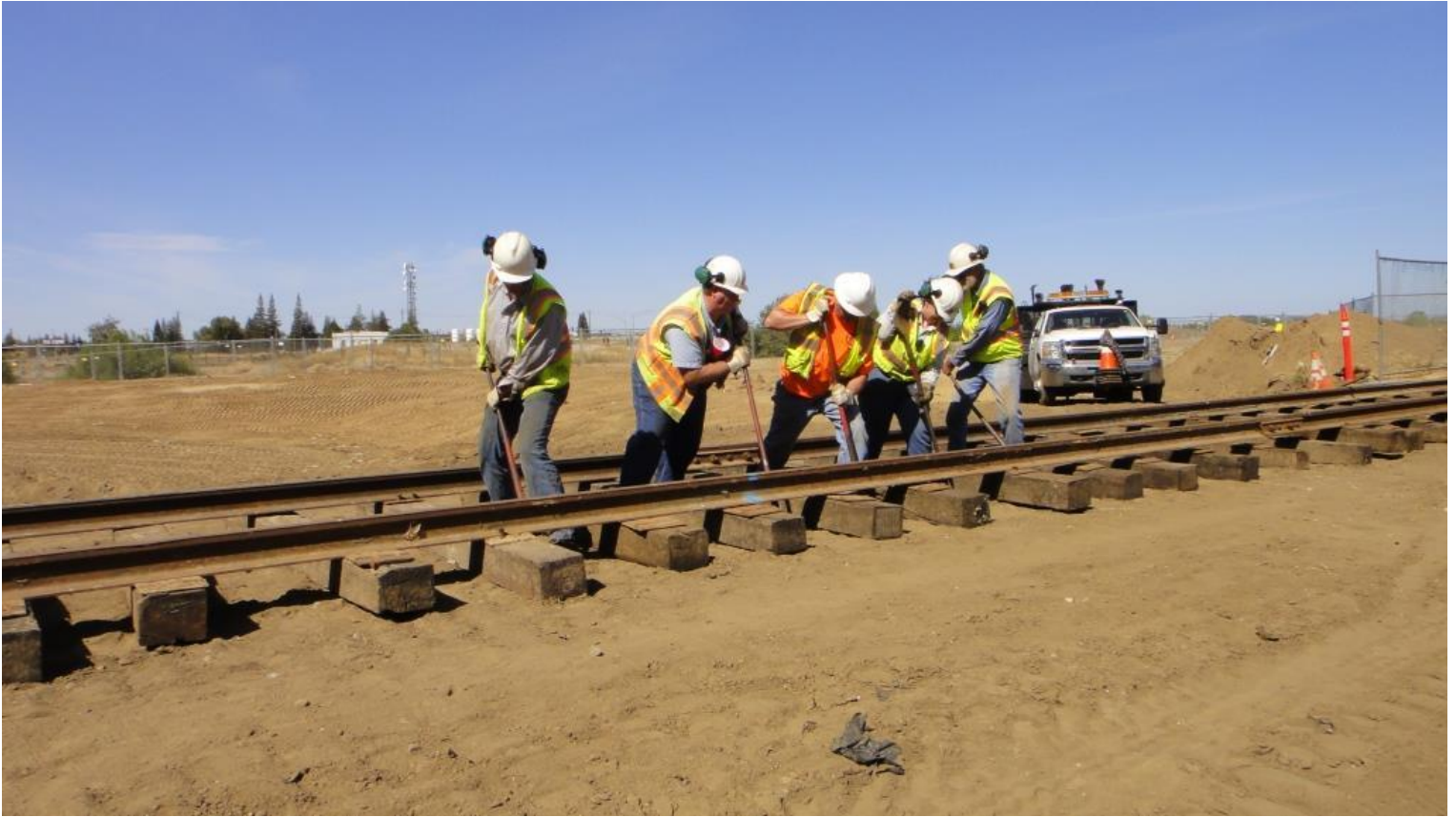
Gandy-dancing! The MOW Team interprets old fashion railroading by using lining-bars in sequence to shove the entire track into alignment
