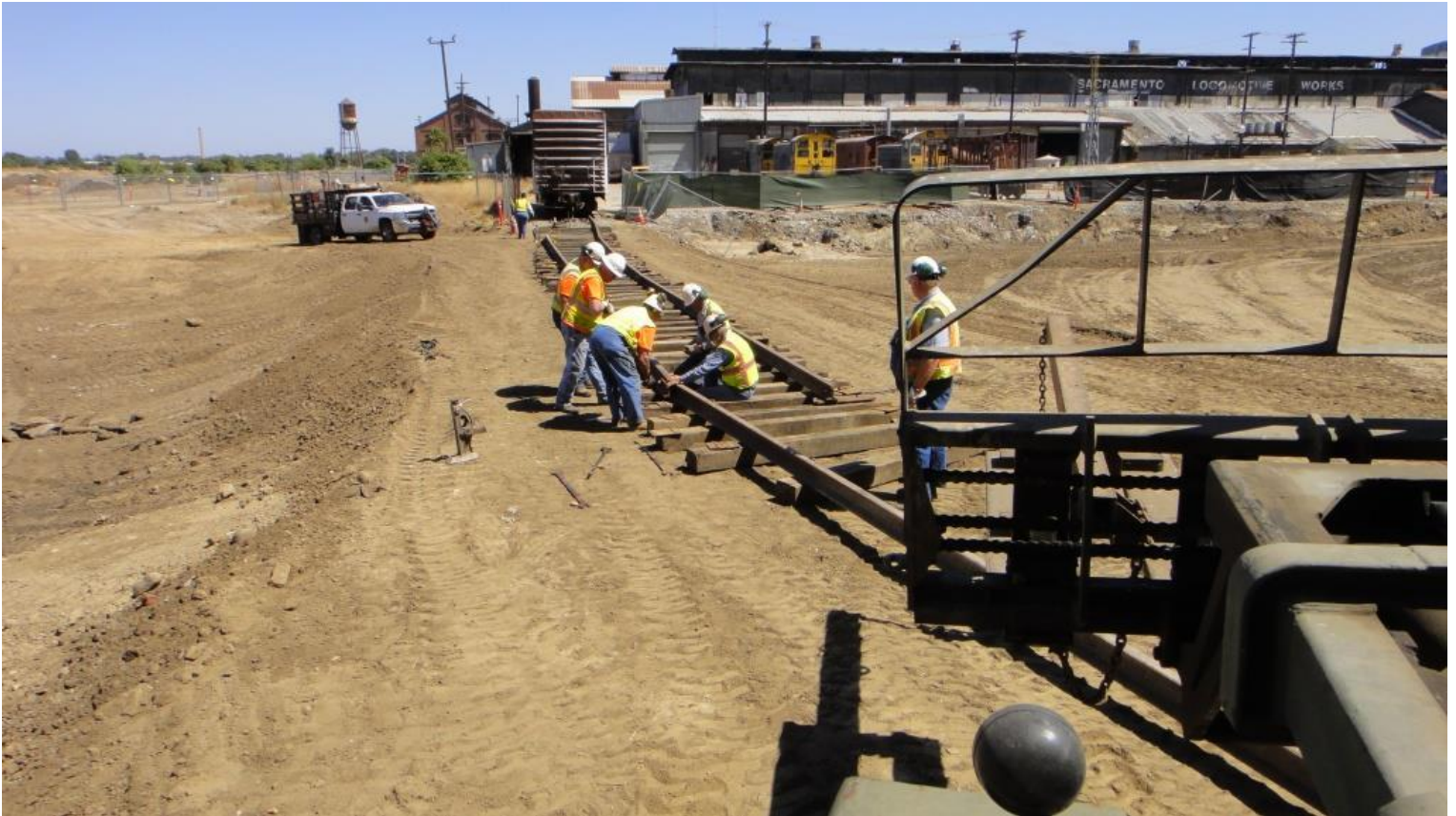
Now for the other side: the Team bolts the rails together which will then be shoved over the rollers by the Green Machine
