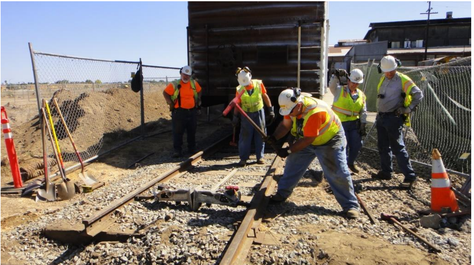
Now in gauge, Mike F. spikes it down
