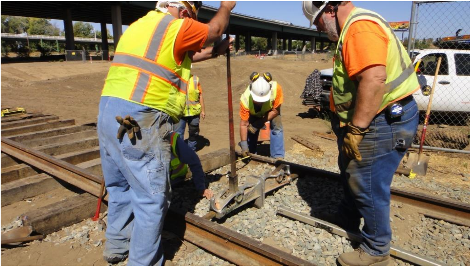
With the rail bolted in place, Mike F., Frank, and Clem gauge it using opposing track-jacks to push the rails apart
