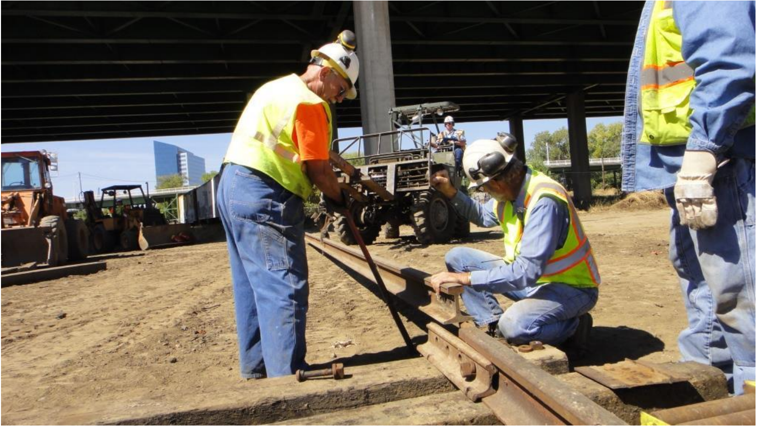
Now for the next rail, Clem guides it with a lining-bar, Alan provides signals to Chris who is maneuvering it into position
