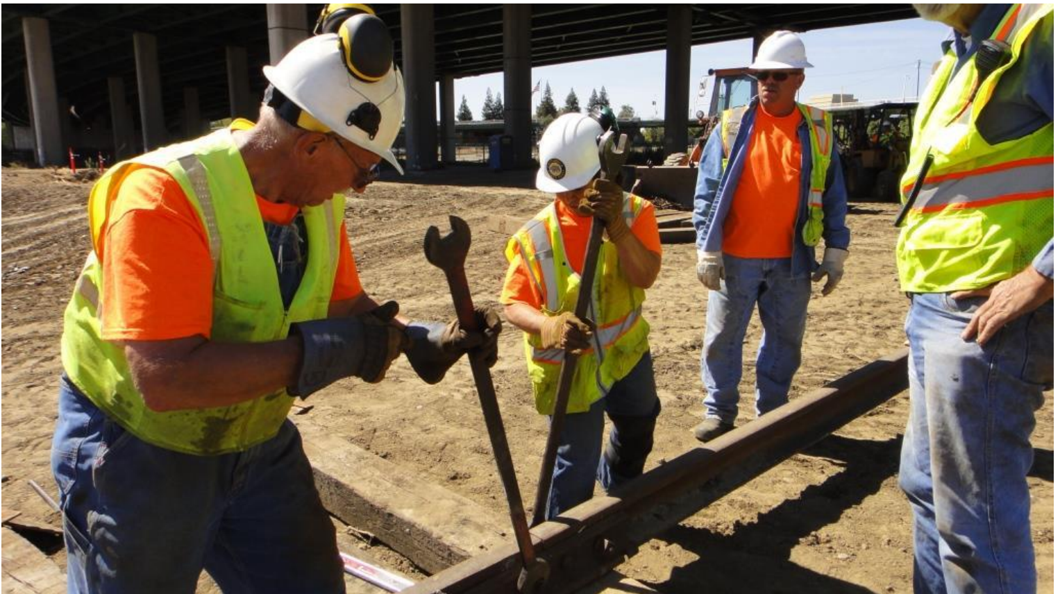
Clem and Pam use track-wrenches to bolt the two rails together
