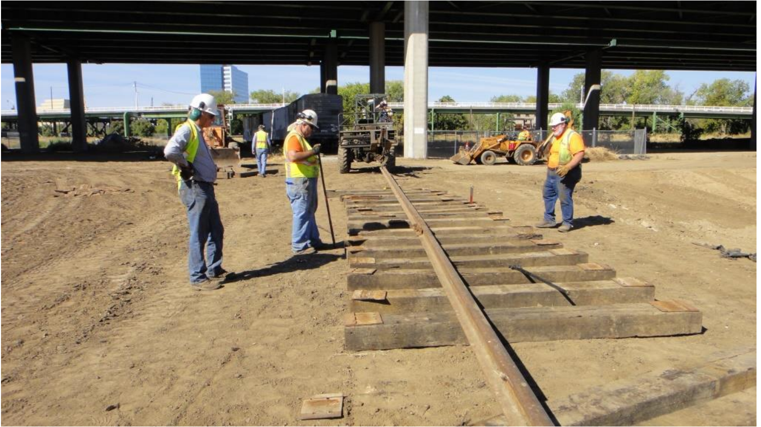
Chris on the Green Machine rolls the rails into position
