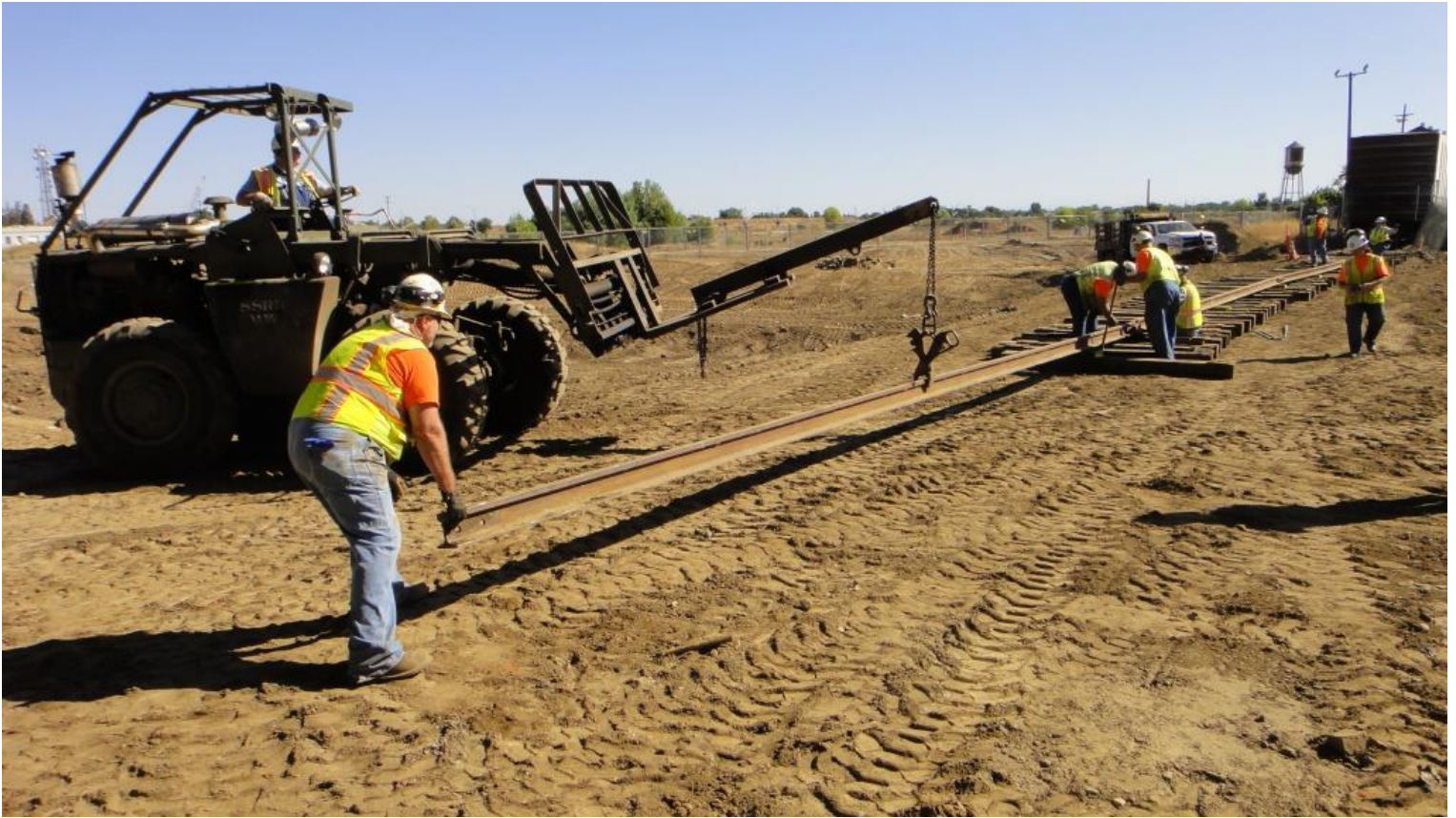
The second rail is brought in. It is bolted to the first then will be rolled into position
