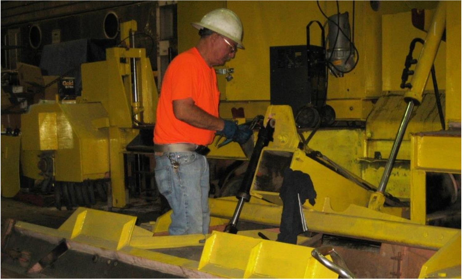
Mike H. reinstalls the repaired hydraulic cylinder on the ballast regulator
